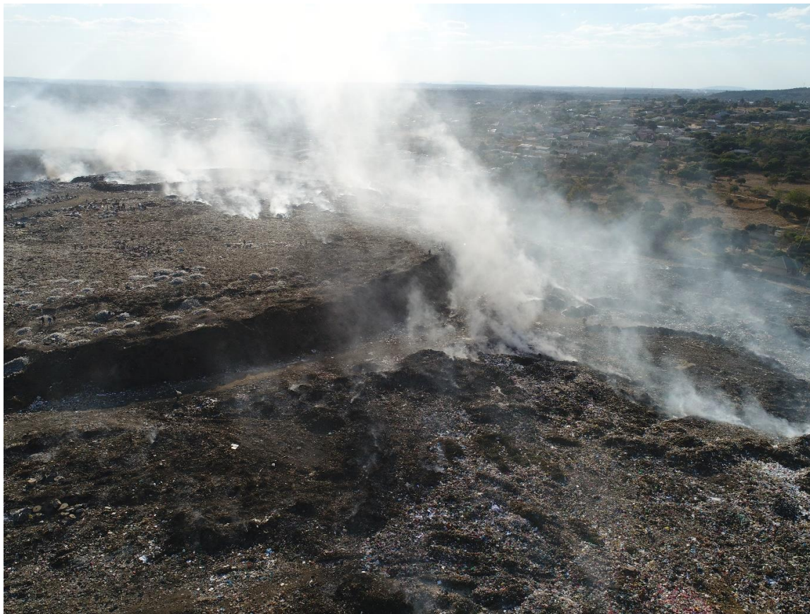
Figure 7. Smoke Plumes from subsurface fires at Chunga landfill resulting from multiple fire focal points across the landfill. The Plume blows primarily west to south west affecting residents of surrounding communities (Aerial Image taken at the landfill site).
